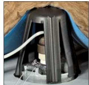
SpotClip-II shown using standard insulation wool.
