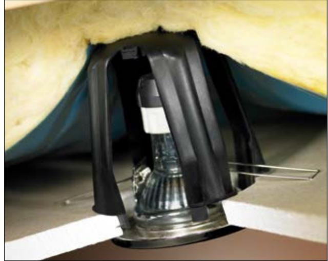
SpotClip-I installed in a dry mortarless construction with insulation wool.
